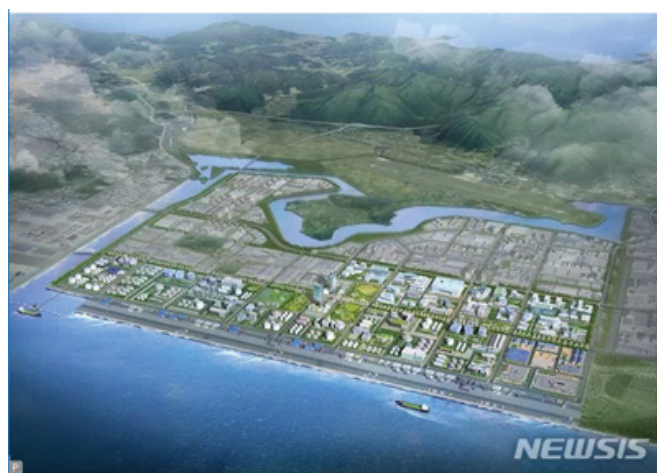
[Gwangyang=Newsis] Bird eye view of Jeonnam Gwangyang Port 3rd-Phase Dredged Spoil Disposal Area Development Project (July 11, 2019)
